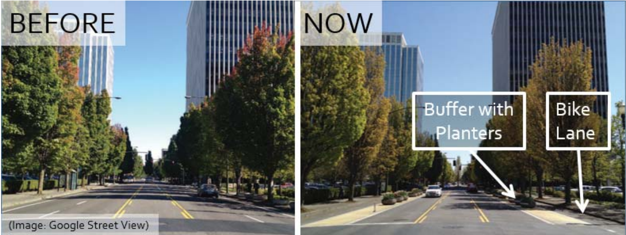
Figure 3-26. NE Multnomah St., Portland, OR, Before and After Installation of Protected Bike Lane
