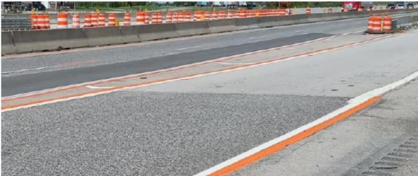
Figure 1 – Initial Installation of Orange Traffic Paint
