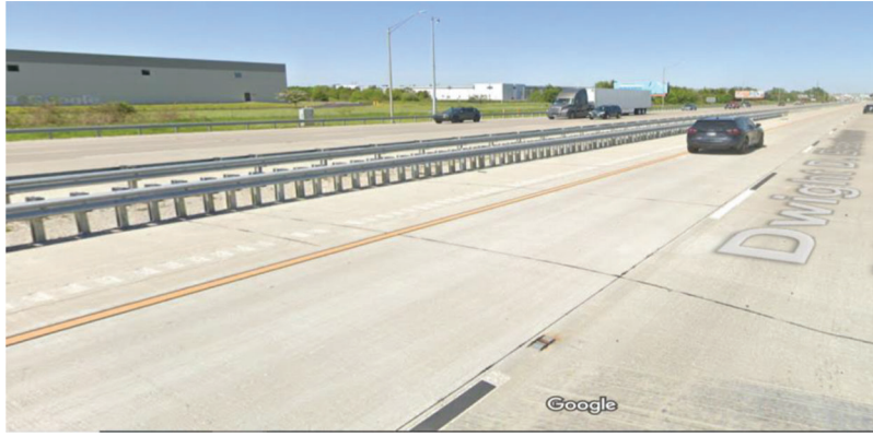
Figure 5.2 Contrast marking I-65 at the I-465 south junction.
