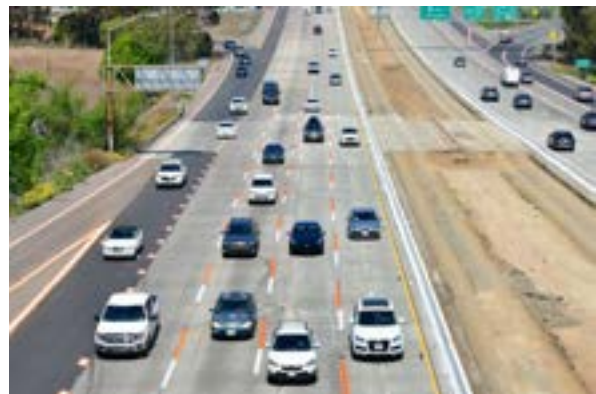
Figure 2. Orange Marking Application on Interstate 5 Southbound
