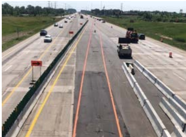
Figure 4. Lane Shift Pavement Markings on Interstate 96
