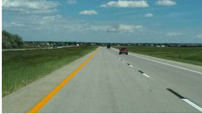
Figure 16. Typical CDOT pavement markings for light-colored concrete surfaces where a 6-inch wide preformed pavement marking tape is used for the centerline skips along with a Lag/Shadow contrast (black) tape marking (Colorado DOT).
