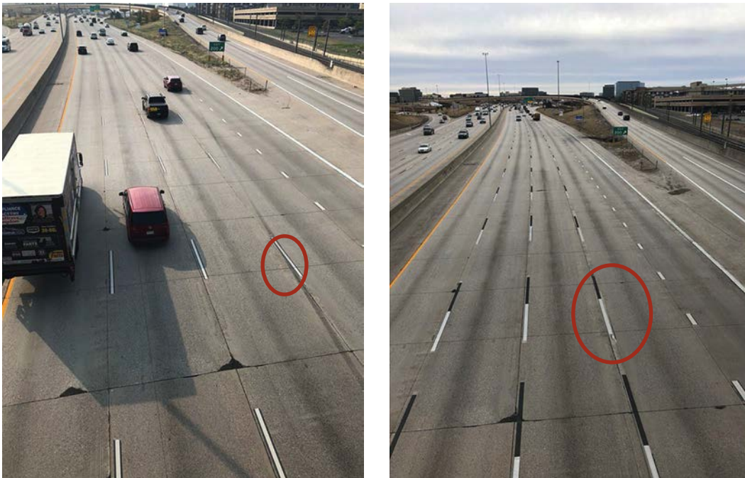
Figure 15. Contrast marking comparison for the same roadway before (left) using 4-inch wide tape with a Bordered contrast style and now (right) 6-inch wide tape using the Lag/Shadow contrast style (Colorado DOT).
