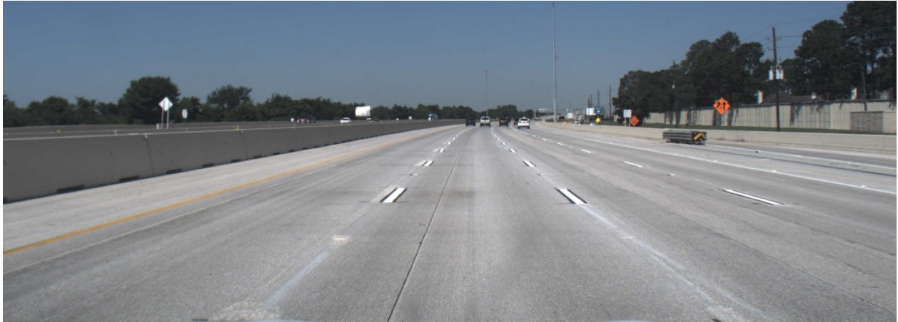
Figure 6. Image of a road segment with white pavement markings with a black border (driving westbound).
