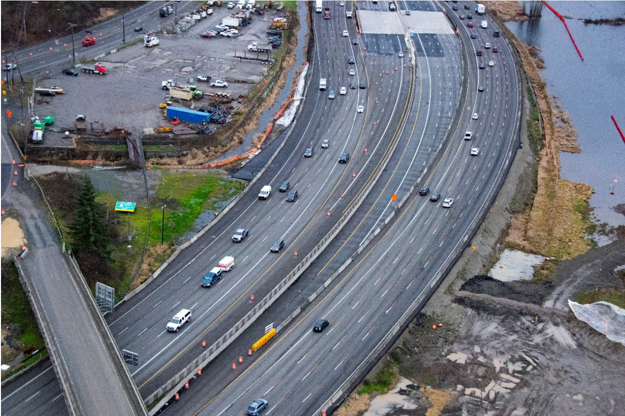
Photo below taken January 2024
