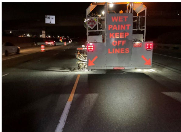
Northbound Interstate 5 orange installation
